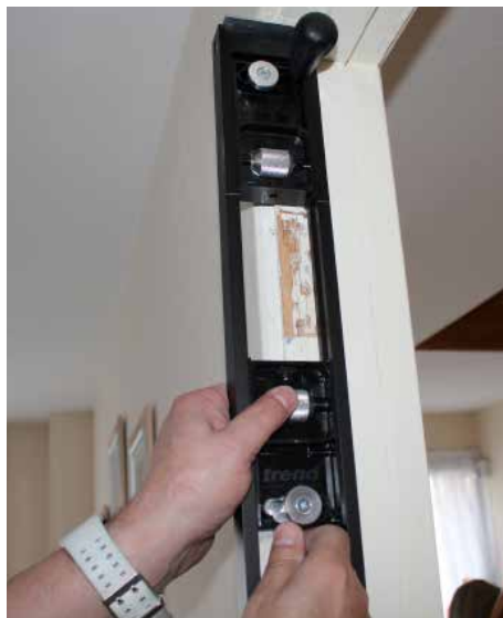
▲ On an existing frame each hinge position is set by sliding the blocks to the correct position
