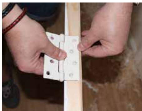
▲ The resulting fit is perfectly flush and crisp
