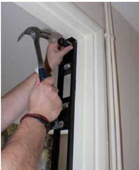
▲ The jig is secured to the door or frame with the supplied bradawls
