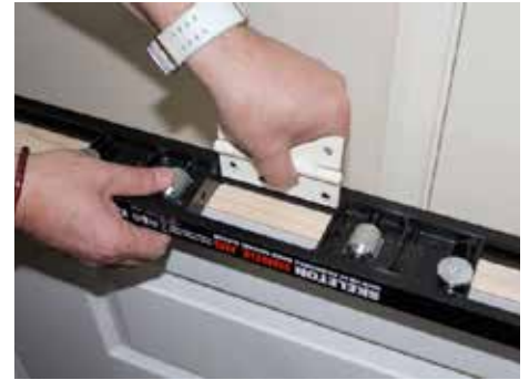
▲ On new work the hinge is used as a gauge and set between the small lips
