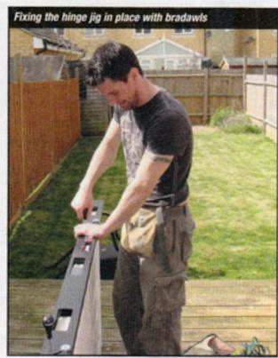
already recessed frames. The first thing to do is to set the width of the recess and this is done by laying one leaf of the hinge on the jig (lining it up with the scribe line on the edge of the jig) and then moving the edge stop up to meet it and then tightening.
