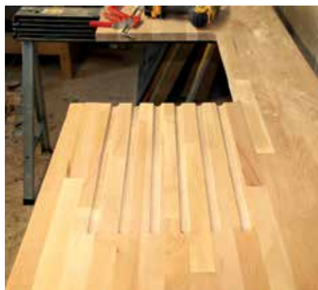
▲ The grooves are clean and consistent with a slight fall
