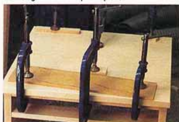
38 Cut the top to overhang the carcass then glue and clamp it in place.
