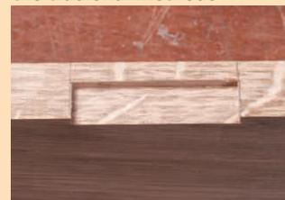
**H**ere is a simple and effective tool to square the corners of routed recesses. Routers are the ideal tool for cutting hinge recesses, but they leave
