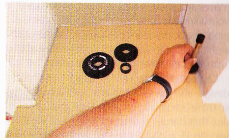
▲ Pic. 1 A loose fitting template is dropped into place and a suitably sized wheel is pushed against the walls and run around them to make an offset mark
