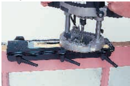
Routing the recess for the faceplate.
