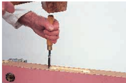
The ends of the recess need squaring off.
