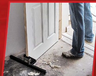
Support to assist fitting door to frame or lining.
