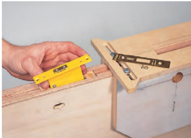
**4.** Before fitting the lock, the spindles and key hole apertures on either face must be cut. To allow easy removal of the lock when fitting it, leave it in the locked position i.e. with the bolt protruding.
